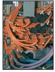
PROFIBUS modules with M23 or M12 connections.
