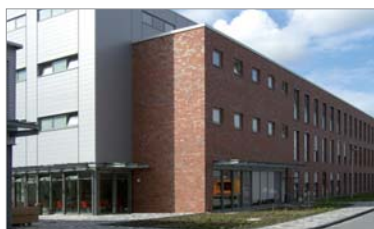
Central office for public services Recklinghausen, Germany Scope of supply: room operation, actor technology, (heating-climate- ventilation, light, sun protection), system components
