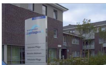
Community & senior citizen centre Lüstringen, Germany Floor space (GFA): 19.200 m 2 Scope of supply: room operation, actor technology (heating-climate- ventilation, light, sun protection)
