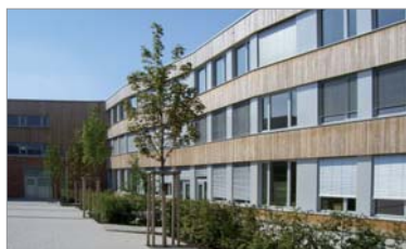
Theobald-Ziegler-School Preungesheim, near Frankfurt / Main, Germany School in passive house technology Scope of supply: room operation, actor technology (licht, sun protection), system components
