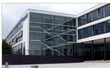
Rhenus Logistik Office building Dortmund, Germany Scope of supply: room operation (heating-climate-ventilation, light, sun protection)
