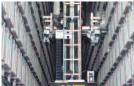
Data transmission to high-bay storage device in conveyor and storage technology
